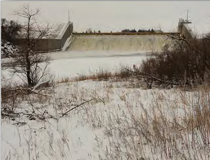
Dickinson Dam, North Dakota, USBR, 1954
